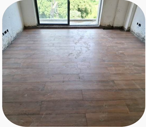
Floor tiling on first floor block D & E
