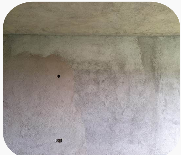
Level 14 plaster in block D & E
