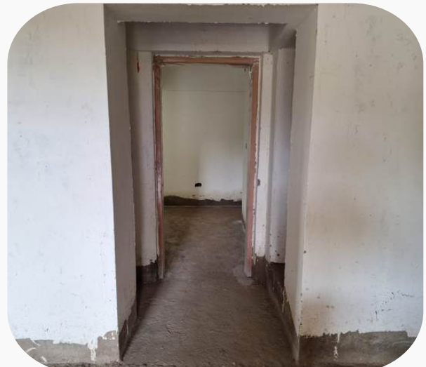
Timber door frames in block D & E
