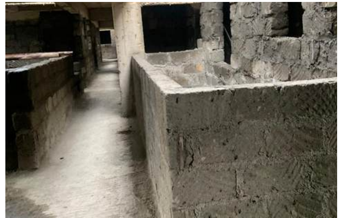
external and internal walling in block C
