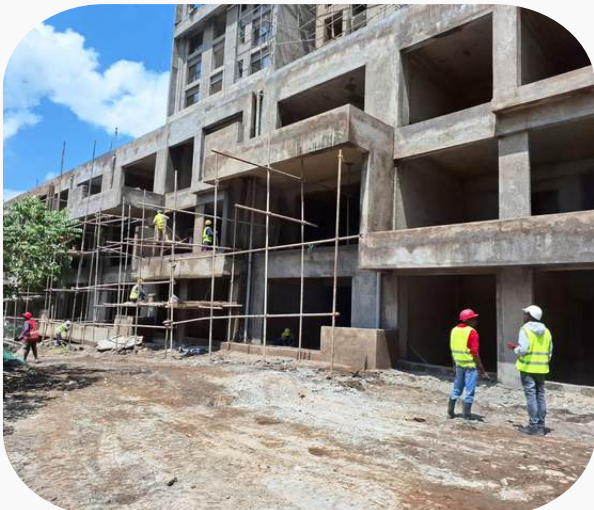
Block D & E river facade external plaster
