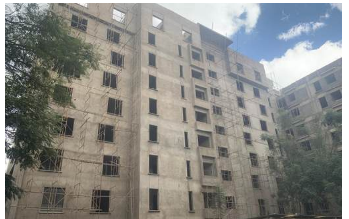
Block C external Plaster 100% complete
