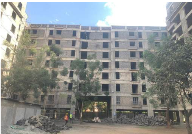
Block B external Plaster Preparation
