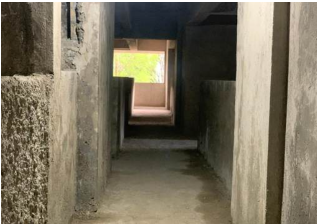
Block C internal Plaster
