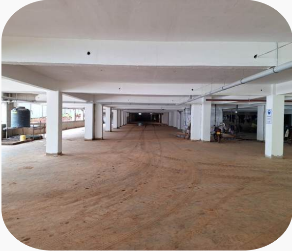
basement parking skimming
