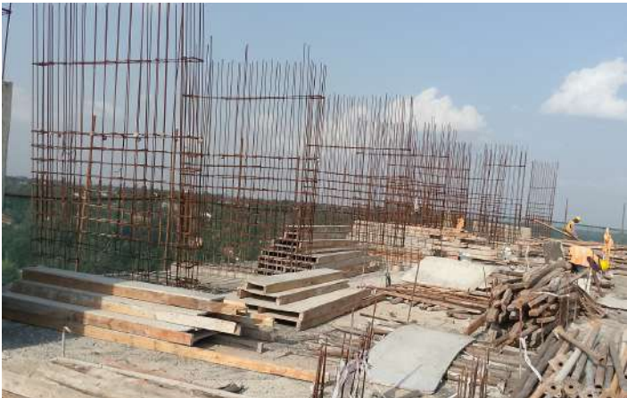
15th-16th Floor Column Reinforcement Works
