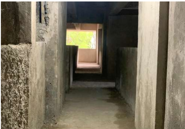
Block C Internal Plaster
