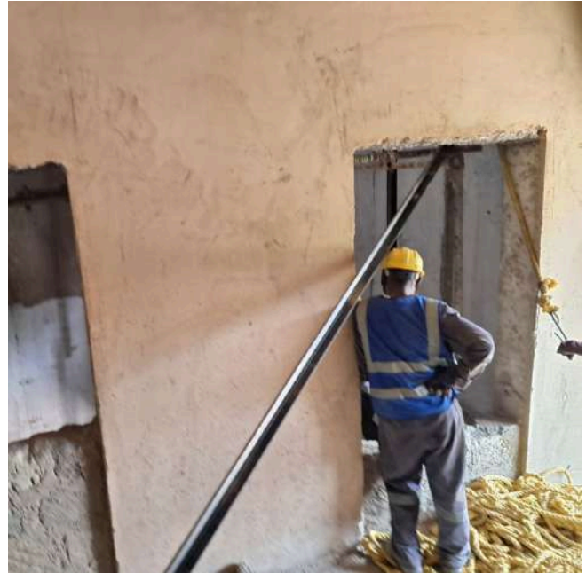
Lift installation in Block D
