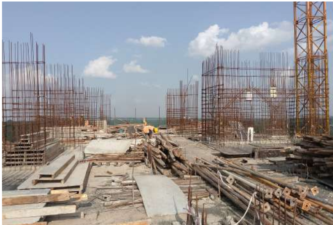
15th-16th Floor Column Reinforcement Works
