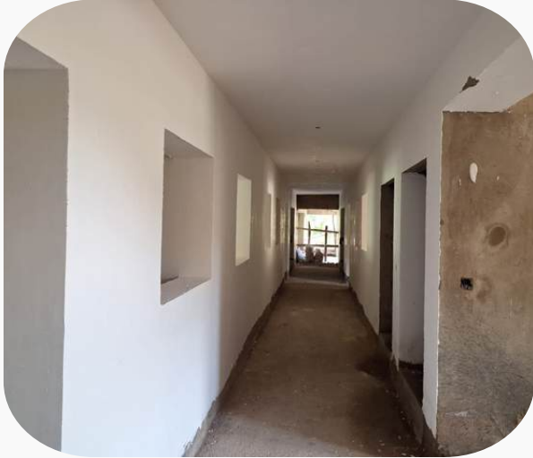
Block D and E corridors skimming
