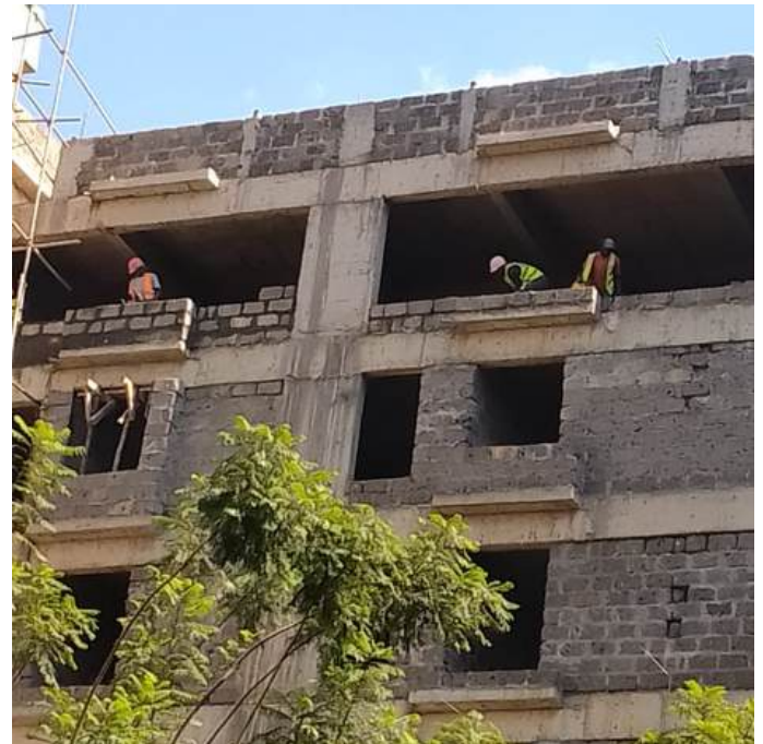
external masonry walling
