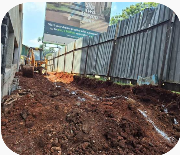
Boundary wall along Limuru Road
