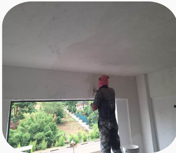
Internal walls skimming
