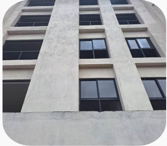
River facade external plaster works
