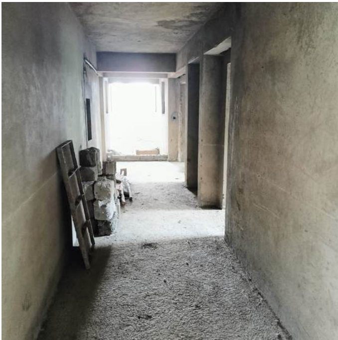
Block C Internal Plaster
