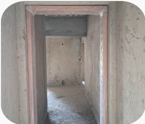
Internal timber door frames installation
