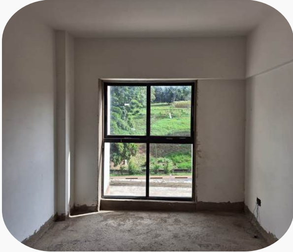
Aluminium windows installation
