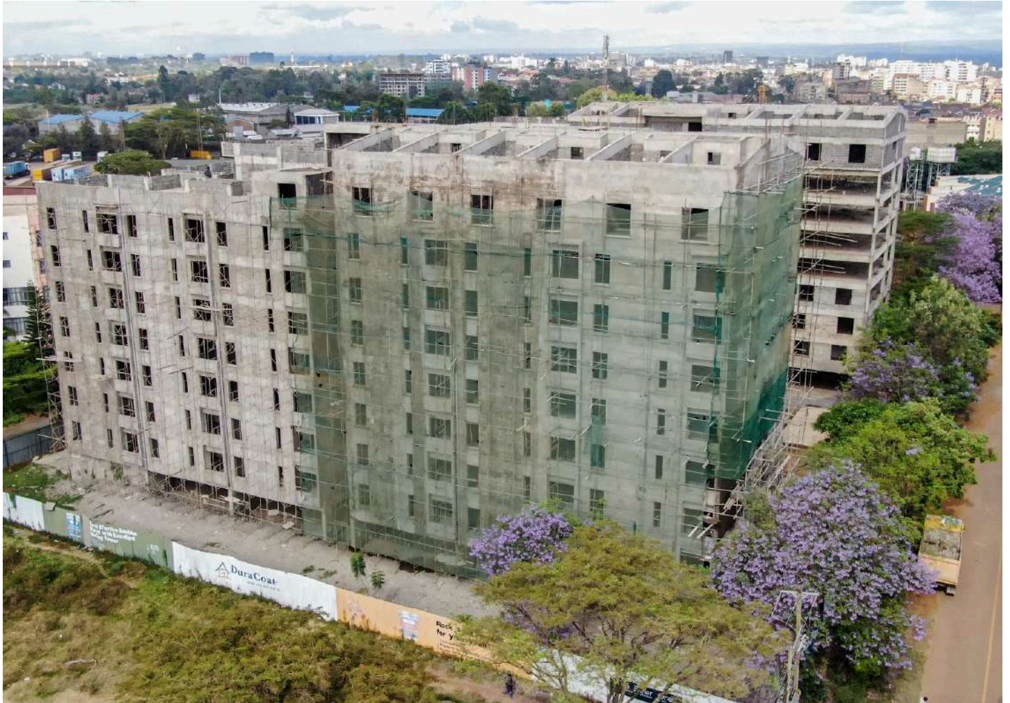
Plaster work on the rear face of Block C
