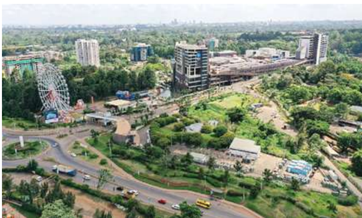
Two Rivers Development featuring the electric substation along the Northern Bypass.
