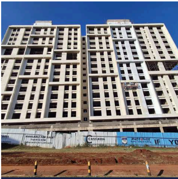
Block D & E view from Limuru Road
