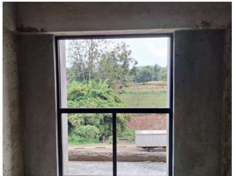
Aluminium window frames installations in Block D, B & E
